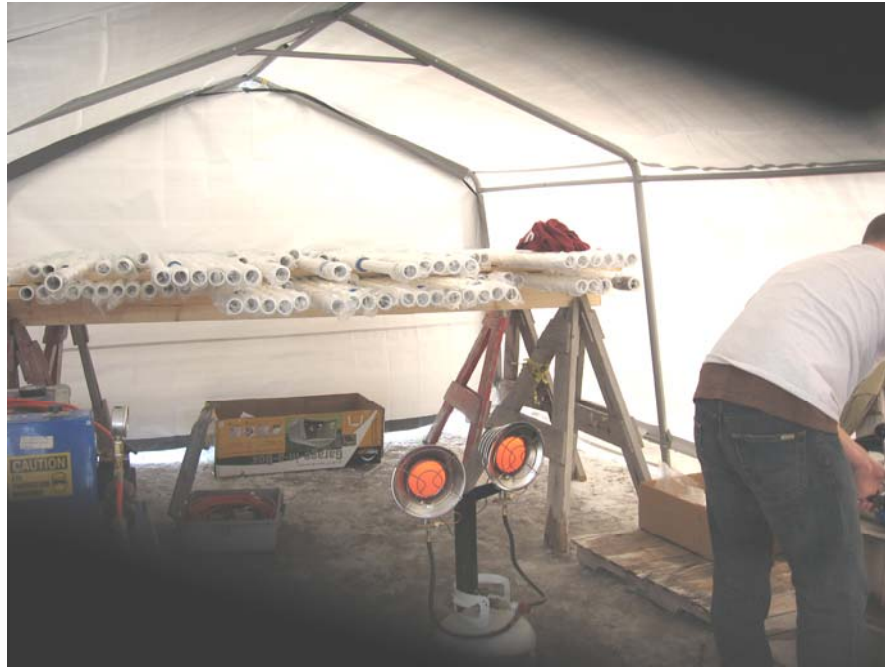
Figure 3 Layout and Installation of MP38 Casing Components at US-8
